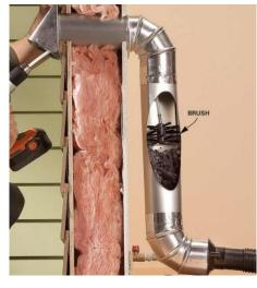
gas or electric. Clean the lint screen after each load and clean the exhaust duct once a year. The Linteater (shown) has an auger brush that attaches to a drill to clean out the ducts.
