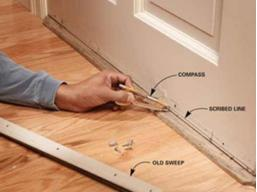
use a scribing tool to extend a mark across the bottom of the door.
