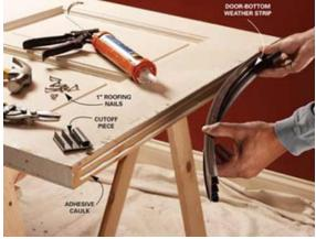
ure the largest gap between the door and the threshold. If the gap is less than 3/8 in., calculate how much you'll have to cut off the bottom to equal 3/8 in. Mark this distance on the door at the point vou meas-
